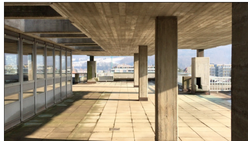
Reto Müller, Potentielle Normaliensammlung, 2017, filmstill [building by architect and sculptor Walter Maria Förderer (*1928)]
